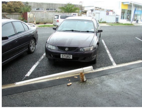
Damage caused by an out-of-control car in Napier Street, Opunake.
